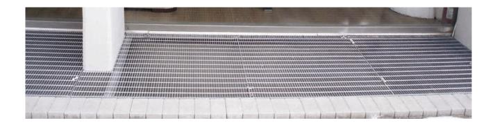
Guardrail open steel flooring consists of flat bars on edge restrained by twisted square or indented round bars forge welded at right angles to give a grating mesh that offers high strength to weight ratio.
